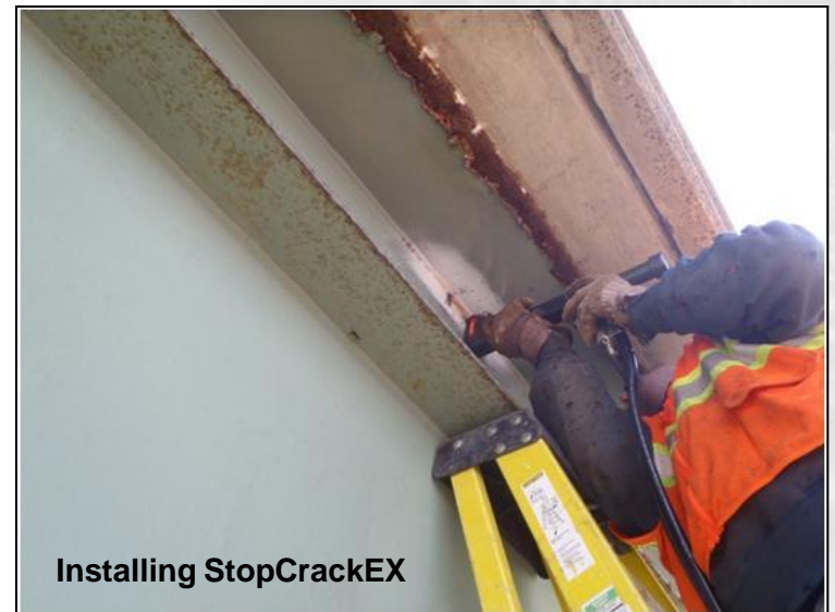
Reaming Drill Stop Hole
