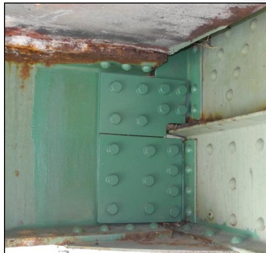
Alternate Doubler Repair
